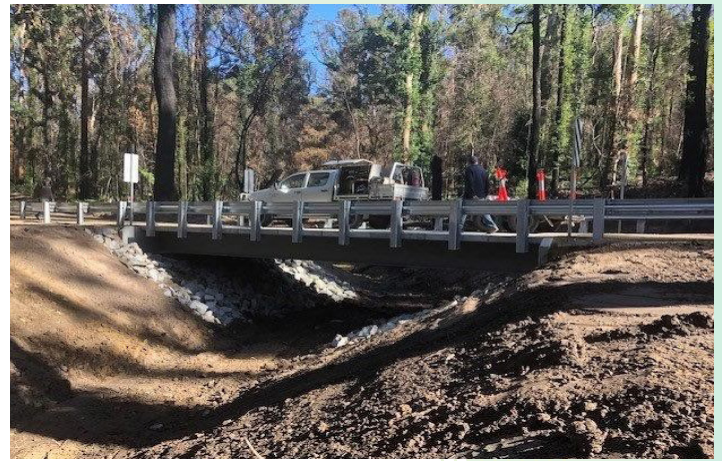
Fairhaven Road Little River Tributary Bridge: after.
