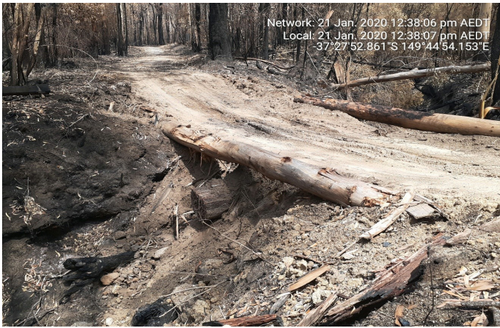
Fairhaven Road Little River Tributary Bridge: before.
